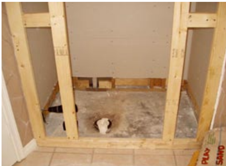
Figure 4. Studs installed sidewise to gain space in shower.
