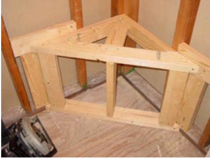
Figure 5. Note the backing blocks at the sides and top.
