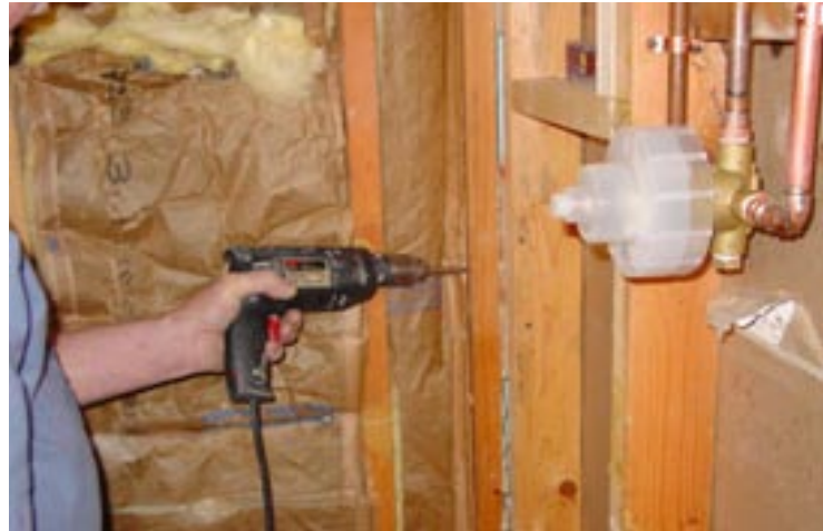
Figure 3. Corner studs are screwed together.
